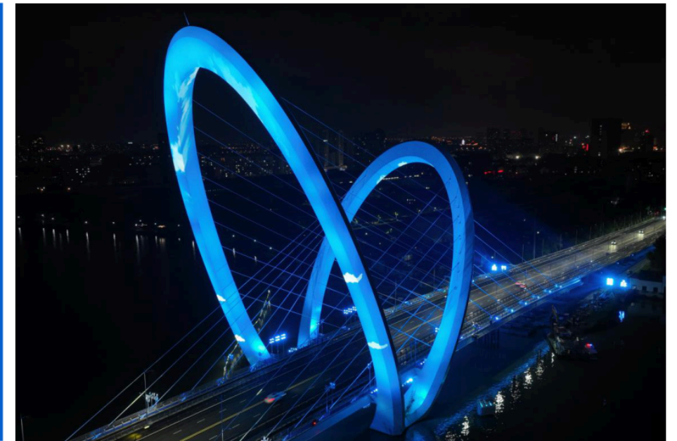
Project: Jiangsu • Zhenchuan Bridge Product: Pattern Light Controller: sunlite-ec
